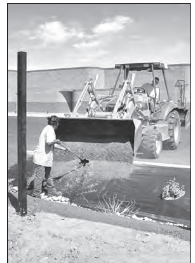
Crews from Martin's Lanscaping laid landscaping cloth and red volcanic cinders in the retention basins, which have drip irrigation systems for the plants and river rock at the bottoms for drainage. QUECHAN NEWS Photos by William Isbell
