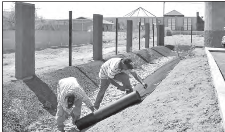
Crews from Martin's Lanscaping laid landscaping cloth and red volcanic cinders in the retention basins, which have drip irrigation systems for the plants and river rock at the bottoms for drainage. QUECHAN NEWS Photos by William Isbell
