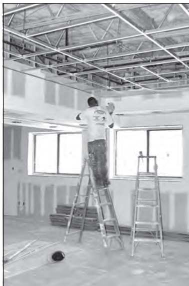
Drywall work and acoustical ceiling installation (at left) were still being done as the tour group made its way through the still unfinished structure. Above on the left, Mr. Brooks points out where stoves and counters will be installed in the front of the industrial kitchen area, while in the top right photo the group moves into the center of the building to take a look at the two-story tall clerestory room that will be used for craft projects, with natural light filtering down from above. At right, a worker finishes up a concrete pier that serves as footing for an outdoor seating area that doubles the size of the dining room when the large doors in back of him are folded open.
