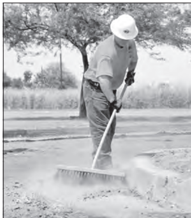
First step was removal of curbing on the south side (at left) where a new spillway into a retention basin will be installed. At right, Don Hamilton of Desert Road Builders sweeps away years of accumulated dust and gravel prior to the start of paving operations in early August.
