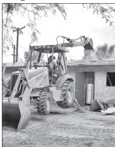
First step (left) is removal of the coolers and roof structure of the homes by Mike Duwyenie on the back hoe. Once the homes are torn down and the foundation is cut into pieces with a jackhammer, Deshane Taylor, Tom Duwyenie and Brandon Durand load the concrete chunks into the backhoe scoop for disposal.
