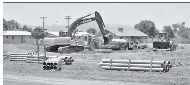
Heavy machinery from Don Peterson Engineering has been on-site, digging trenches and putting water and sewer lines in place, all under the watchful eyes of a Tribal Monitor.
