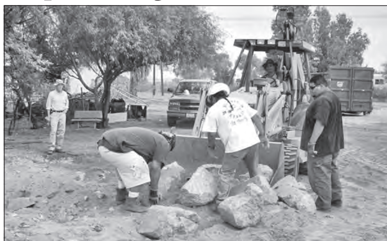
First step (left) is removal of the coolers and roof structure of the homes by Mike Duwyenie on the back hoe. Once the homes are torn down and the foundation is cut into pieces with a jackhammer, Deshane Taylor, Tom Duwyenie and Brandon Durand load the concrete chunks into the backhoe scoop for disposal.
