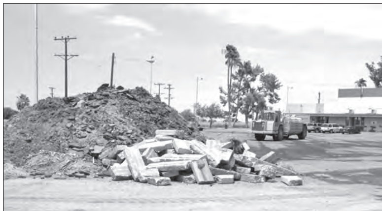
First step was removal of curbing on the south side (at left) where a new spillway into a retention basin will be installed. At right, Don Hamilton of Desert Road Builders sweeps away years of accumulated dust and gravel prior to the start of paving operations in early August.
