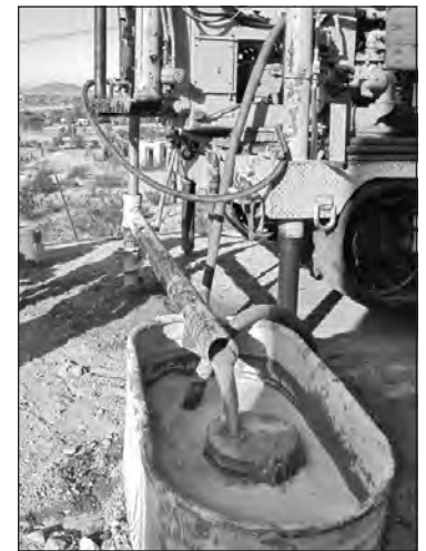
Drilling crew from GSI Drilling carefully monitors their progress on the west side of the water tower, at left. Water used as a lubricant for drilling into the granite bedrock on Indian Hill is recycled throughout the process. QUECHAN NEWS Photos by William Isbell
