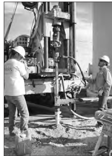
Drilling crew from GSI Drilling carefully monitors their progress on the west side of the water tower, at left. Water used as a lubricant for drilling into the granite bedrock on Indian Hill is recycled throughout the process. QUECHAN NEWS Photos by William Isbell
