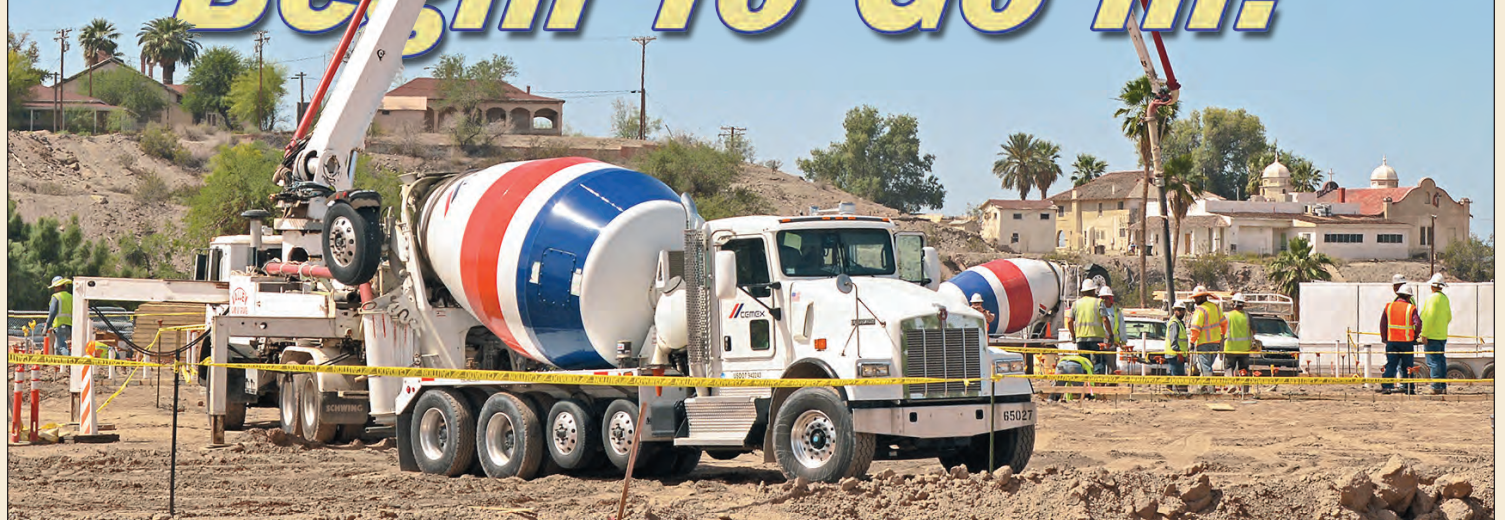
Concrete began to flow into the footings for the new Fort Yuma Health Care Center's Building A on Thursday, May 5th, under the watchful eye of the on-site superintendents working for Pilkington Construction, the general contractor on the 20 month project. Quechan News Photo by William Isbell
