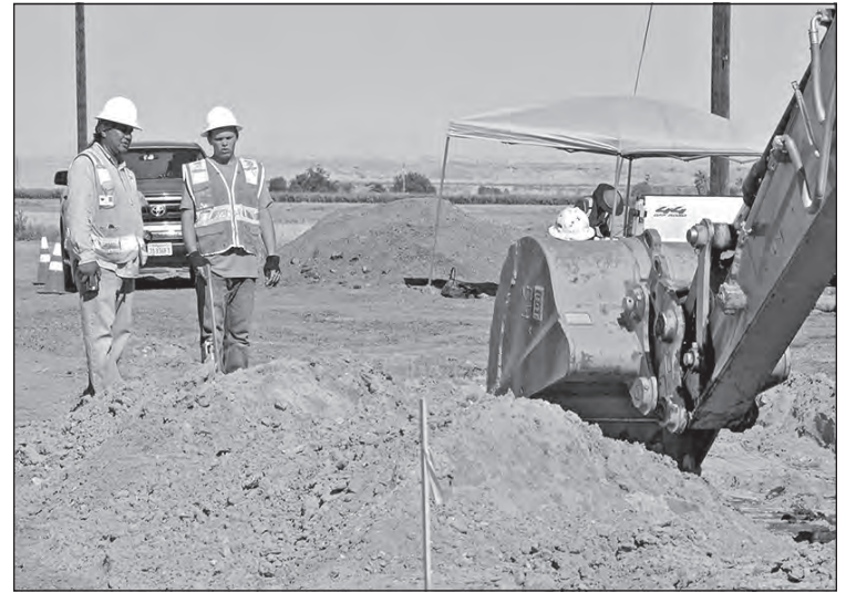
The first phase of the project began on June 22nd, with Pyramid Construction removing the most deteriorated pavement between First and Foster Roads all the way down to the dirt below. Once that area is brought back up to the same level as the remainder of Arnold Road (using a gravel base course), the entire road will be repaved from Picacho to Foster. A Tribal monitor is on the project to observe all digging. QUECHAN NEWS Photos by William Isbell
