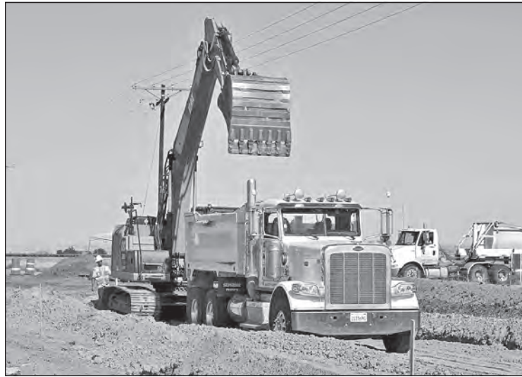
The first phase of the project began on June 22nd, with Pyramid Construction removing the most deteriorated pavement between First and Foster Roads all the way down to the dirt below. Once that area is brought back up to the same level as the remainder of Arnold Road (using a gravel base course), the entire road will be repaved from Picacho to Foster. A Tribal monitor is on the project to observe all digging. QUECHAN NEWS Photos by William Isbell
