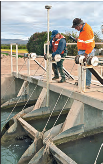
Every feature of the gates, canals and support structures are measured in order to develop a 3-D computer model of how the water flows within the Bard Water District.
