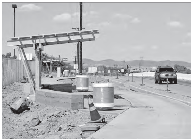
A crew from CalTrans contractor rsm 2 Constructors, Inc. is installing new sidewalks, handicapped ramps, shade structures with informational kiosks and decorative safety lighting. Q NEWS Photo by William Isbell
