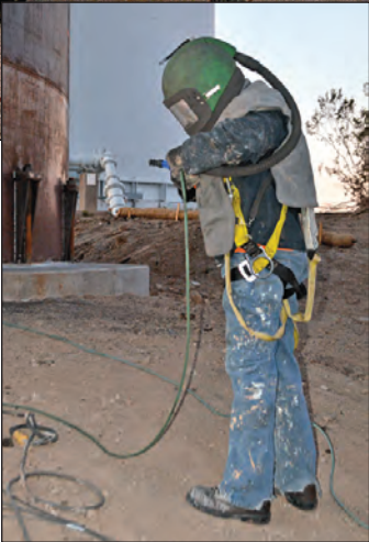
A painter prepares to attach the fresh air supply line to his helmet just before entering the water tank for a long hard day of sandblasting. QUECHAN NEWS Photos by William Isbell
