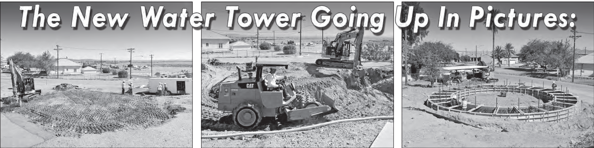
Work on the new water tower began with site preparation, digging down to the proper level and compacting the soil to increase it's density. A 6 foot thick ring 40 feet in diameter was then dug down around the perimeter, to set the marine grade plywood concrete footing forms in place. All the while, the entire footing area was watered down and further compacted. Once the plywood forms were in place, steel rebar reinforcement mesh was placed inside the forms and wired securely into place.
