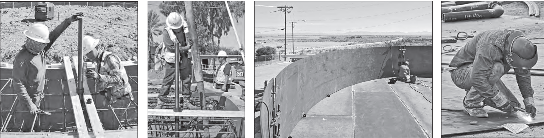
Twenty four threaded steel rods over 6 feet long and 3 inches in diameter were carefully positioned, evenly spaced along the centerline of the foundation ring. Once the steel reinforcements were in place, high strength concrete was pumped into the forms and allowed to cure for a week before the 3/8th inch thick steel flooring panels were welded in place. The tub ring was then welded together and bolted down, with hatches and outlets for pipes later cut through and installed. Steel plate for the rings have attachment points welded on.
