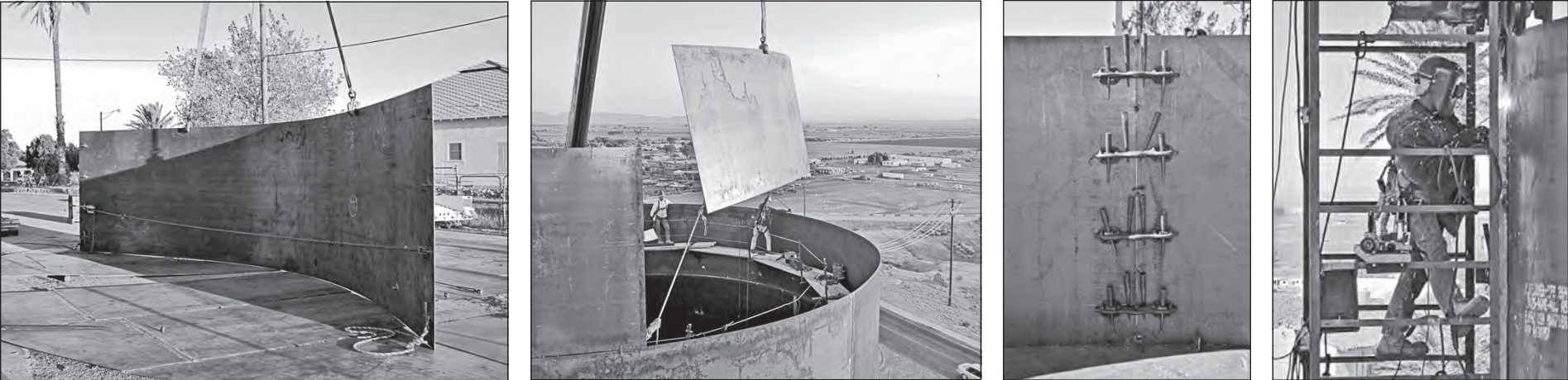
The ring plates are curved by attaching a chain and cinching it down with a "come along", until it takes the proper shape. The plates are then lifted into position by the crane operator, as workers inside the tank guide them into place by hand. They raise their steel framed wooden walkway once each level is completed. Attachment points previously welded on have steel clip rings and wedges driven into them by hand, hammering the ring into a perfectly round shape. Steel cages on rollers allow the welders to move about the exterior.
