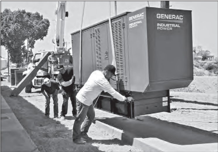
Dave Amos of Sellers' Crane Service lowers a 35KW diesel generator onto a pad near the Tribal Administration Office. Walt Brooks, the Quechan Tribe's construction coordinator watches Daniel Albert and Saul Nuñez of GenTech guide it into place.
