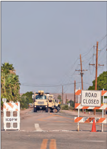
Over two dozen high voltage power poles went down along Araz Road west of Third Avenue.
