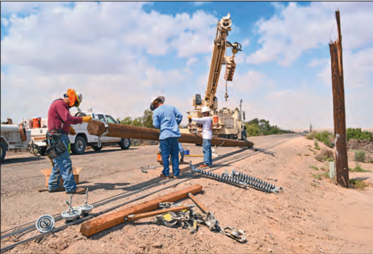
At least 8 construction crews were hard at work early Friday morning, cleaning up the downed power poles. Once that was done, they got to work on custom building new poles and getting the lines back up.
