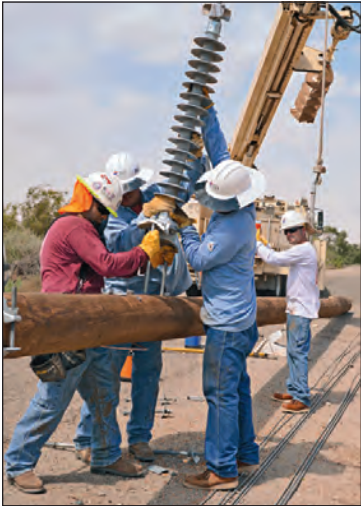
Brand new insulators and cross-arms had to be installed by hand on each new high voltage line.
