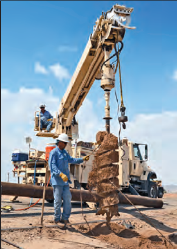
The stumps of old poles had to be drilled out of the ground before the replacements went in.
