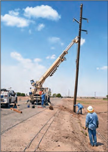
The auger trucks also have a claw on the boom to lift the finished poles and put them in place.
