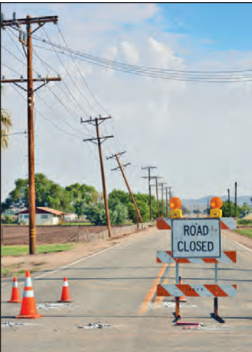
Traffic along Picacho Road was closed to traffic, with dangerous high voltage lines hanging loose.
