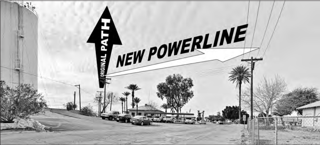
Here is the new powerline after installation: the route now takes a northward jog across the roadway by the Police Station. The original path (black arrow) crossed directly through the planned water tower's space.
