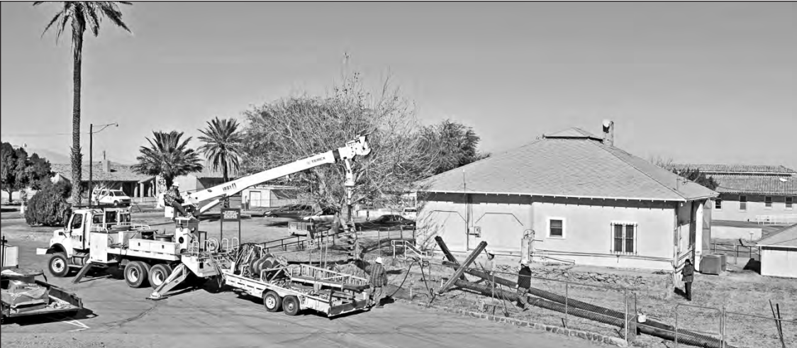
A construction crew from Irby Construction of Jackson, Mississippi was here over the second week of January, drilling holes, installing new power poles and moving the powerlines on Indian Hill. The project was preparing the area to the southeast of the Quechan Police Department for the installation of a second 780,000 gallon water tank later this spring. At left (above) the crew drills a 7 foot deep hole just inside the fence at the IHS main office, then pulls the auger (at right) to shake off the dirt before starting a second pass on the hole.
