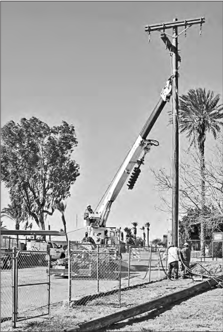
The crew carefully aligned each pole once the drilling machine operator lifted them into place. A large pole with a hook is used to grasp the pole and bring the crossarms into alignment with the route the wire will follow, and the hole is then backfilled and tamped down solid.
