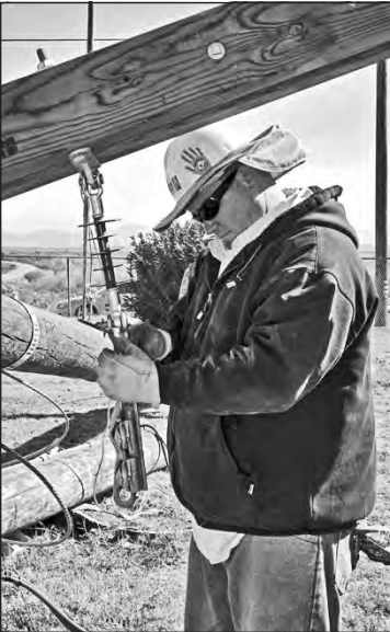
A worker placed wire guides on the insulators just before each lift.
