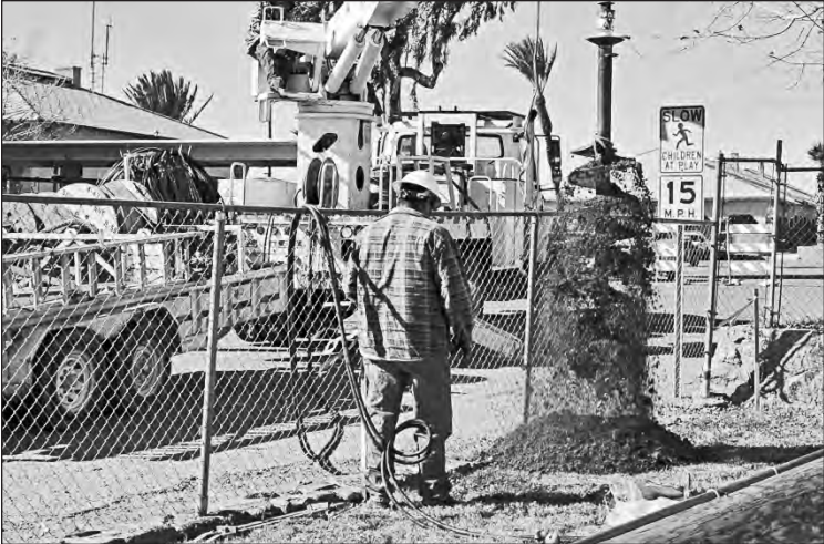
A construction crew from Irby Construction of Jackson, Mississippi was here over the second week of January, drilling holes, installing new power poles and moving the powerlines on Indian Hill. The project was preparing the area to the southeast of the Quechan Police Department for the installation of a second 780,000 gallon water tank later this spring. At left (above) the crew drills a 7 foot deep hole just inside the fence at the IHS main office, then pulls the auger (at right) to shake off the dirt before starting a second pass on the hole.
