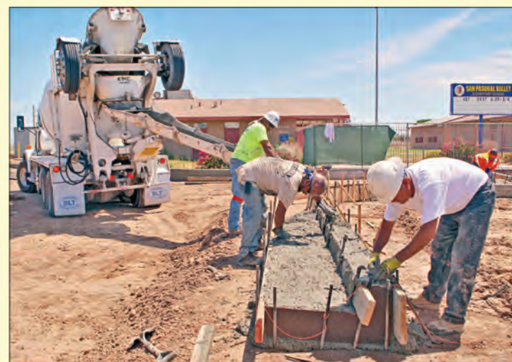
Team C Construction employees Tomas Romero, Jacinto Piña and José Saravia (in the foreground) from El Cajon work on pouring and smoothing new curbs for an all new driveway going in north of the elementary school office.
