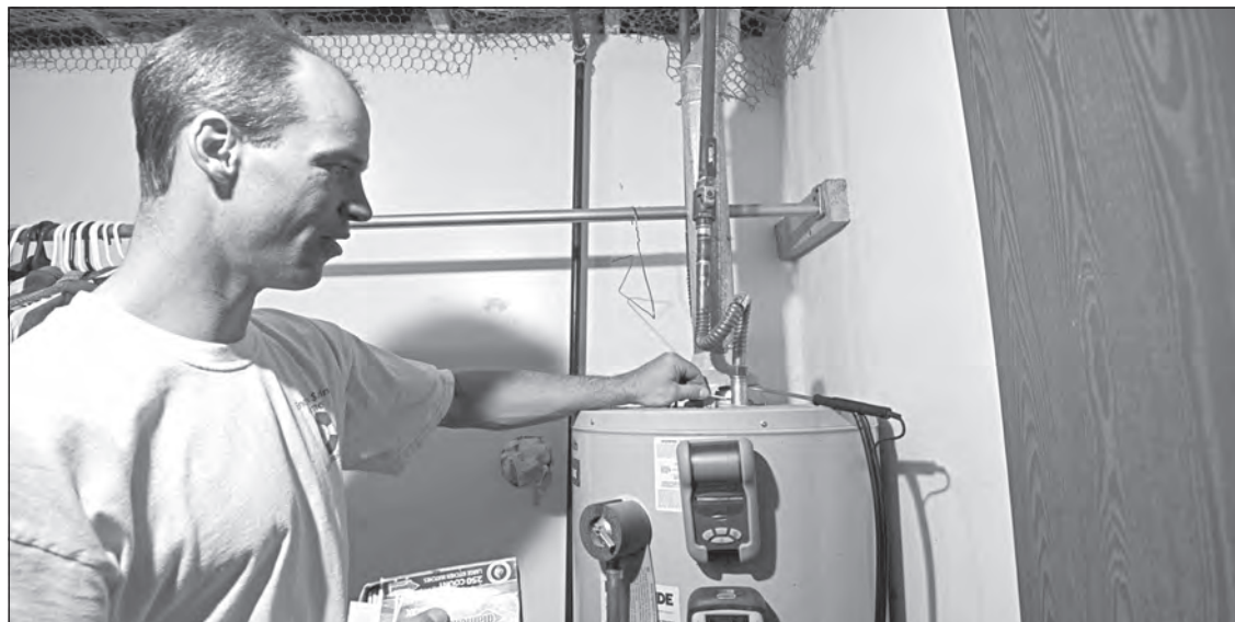
Contractors with the Weatherization Assistance Program will perform an energy audit before beginning the work, to determine what is most in need of an efficiency upgrade. Campesinos Unidos, a contractor from El Centro, will be performing the majority of the work under the program this year. D.O.E. Photo by Dennis Schroeder, NREL
