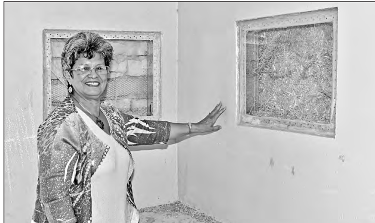
Carver Elementary school secretary Lucille Torres points out the windows left inside the school's kindergarten playhouse. The windows show details of the straw bale construction methods used by the YPIC Youth Build crew Rose Phipps was a part of. QUECHAN NEWS Photos by William Isbell
