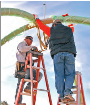
Hector Corral prepares to bolt two arches together as his boss holds things steady.
