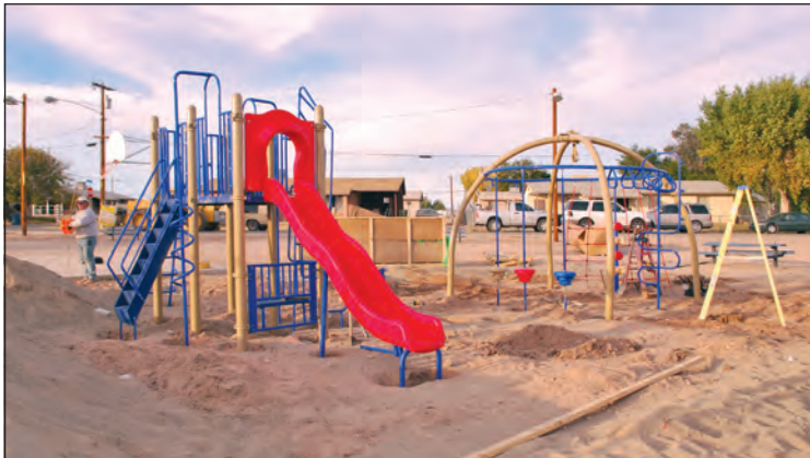
All of the new equipment was installed near the current basketball court. Each outdoor gym structure is held in place with concrete footings, buried at least 30 inches deep, and surrounded by soft sand.
