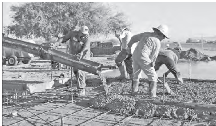
Workers quickly spread and smooth concrete as it pours from the back of a cement mixer, laying the foundation pad of the new Utilities Maintenance Shop below Indian Hill. QUECHAN NEWS Photo by William Isbell
