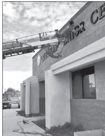
Jordan Bowers of Sign Masters puts the finishing touches on the new Quechan Senior Center sign, installed January 7th.
