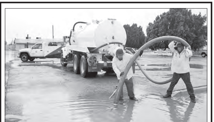
Eddie Vanegas and Mike Duran of the Quechan Work Force team up to siphon water out of a low spot on Quechan Drive during last week's inundation. Other crews from both Quechan Utilities and Facilities were also out at the same time, trying to limit damage during the recent rains. QUECHAN NEWS Photo by William Isbell
