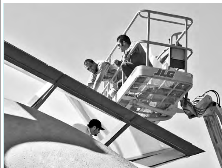
A crew from Sign Masters in Yuma spent a couple of days in late October replacing the plexiglass facets of the huge diamond ring over the entrance to the Paradise Casino. Supervisor J. C. Garcia (inside the diamond) helped Jason Leinbach and Gordon Bowers (on the lift) measure, cut and install 32 sheets of Thermaglass multi-wall polycarbonate in place of the original covering that was installed when the Casino first opened 13 years ago. QUECHAN NEWS Photo by William Isbell
