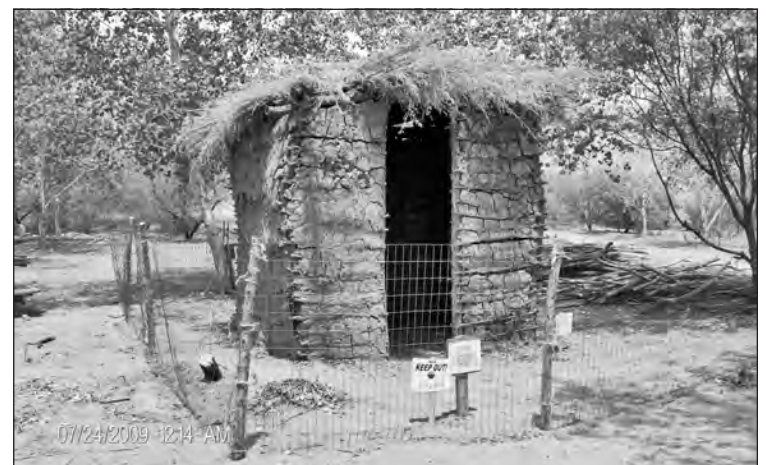
Once repairs were completed , fencing and "No Trespassing" signs were posted to keep people out of the area.
