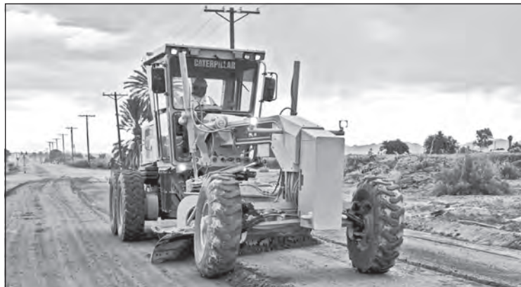
A road grader resurfaces Indian Route 10 (Miguel Road), just one of many roads getting some attention this summer. Photo by William Isbell
