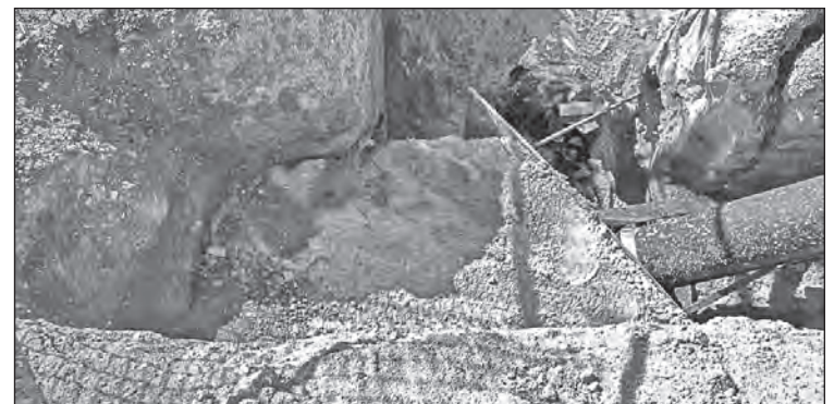
Thrust blocks are solid, heavy blocks of concrete poured in place at the outside corners of high pressure pipe junctions. The weight of the blocks anchor the pipes in place, and prevent the pipes from shifting due to pressure changes when the pumps first turn on.
