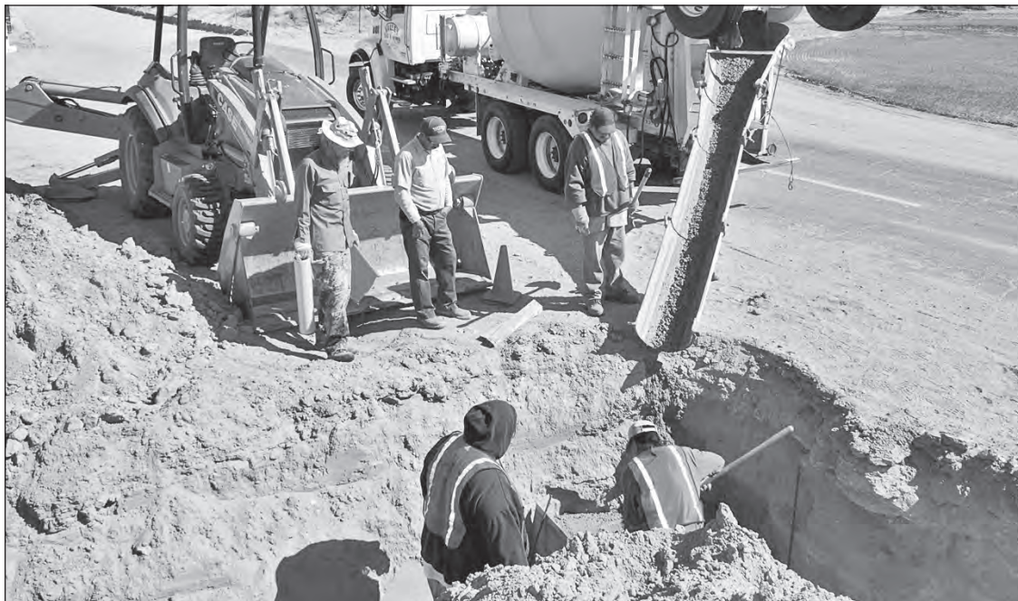
Bill Hirt, Special Project Coordinator for the Quechan Tribe waits next to the delivery driver for Valley Sand and Gravel, watching Tom Duwyenie (next to concrete chute), DeShayne Taylor and Mike Duwyenie (in the hole) finish leveling off the pour into a concrete form for a thrust block. QUECHAN NEWS Photos by William Isbell
