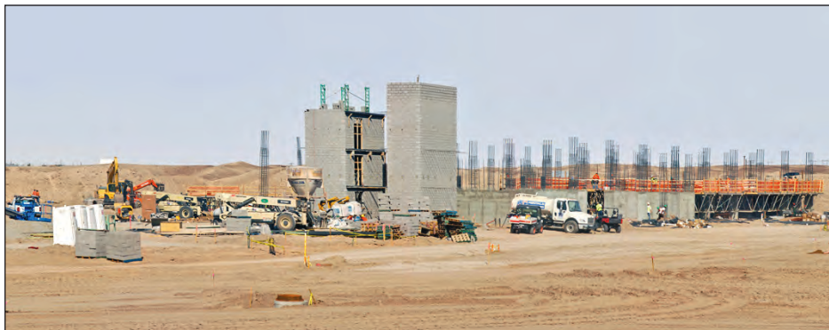
By March 2008 the elevator towers were going up and the foundation was in for the Hotel wing. Things would move more rapidly once the concrete for the walls was being poured.
