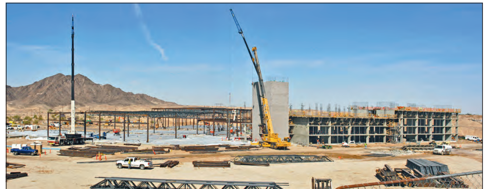
Framing of the Casino and Pipa Event Center shot into the sky in this view taken only 6 weeks later. ROEL began to overlap work shifts to keep things on-track during the summer.
