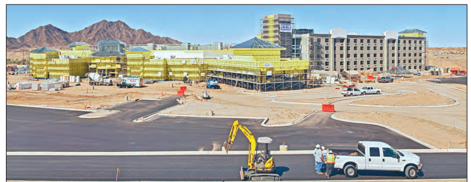
A scant four months later, with 4 shifts starting 2 hours apart every evening, the entire building is enclosed, paving begun and the air conditioning is installed and working.
