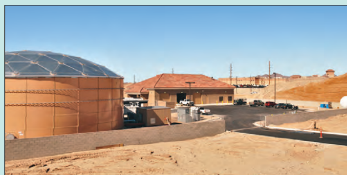
The adjacent water storage and treatment facility is completed and begins operation, completing its first shake-down run and receiving certification to operate by the end of January.
