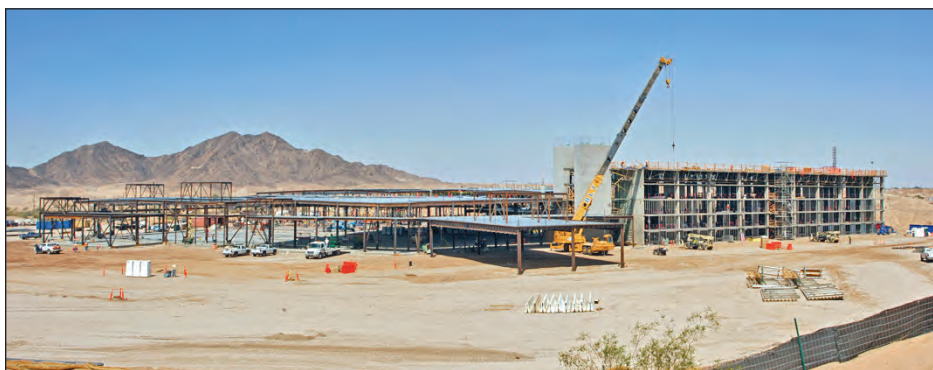
By June, the porte-cochère at the center of both wings extends out over the valet entrance, and all five floors of the Hotel are in place, prior to the walls being erected.
