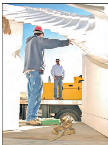
Mike Matthews spent a few minutes making sure the crane operator had everything ready to go.
