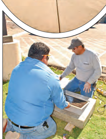
Meanwhile, D & K Concrete men set the bronze dedication plaque into its stone base.
