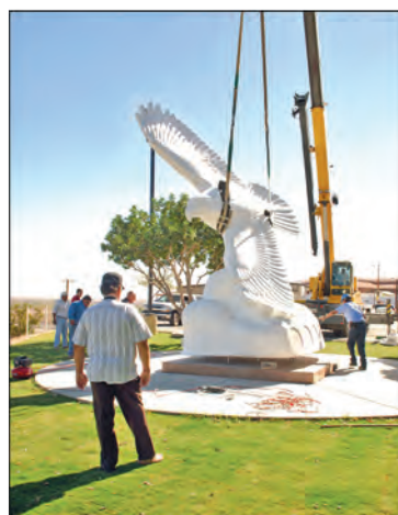
Once the holes were drilled, the Eagle was carefully lowered into position and grouted into place.
