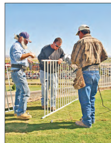
Finally, a safety rail fence was put in place at the edge of the hill by an All Valley Fencing crew.
