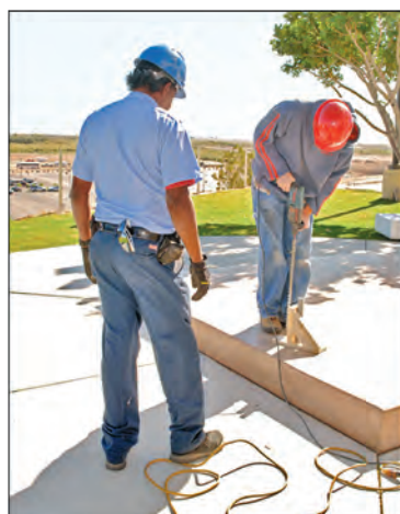
Lead Sculptor Mike Matthews begins to drill holes for the locating pins, as Lonnie Gilmore watches.
