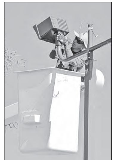
A Westmoor Electric employee installs the first of three lights atop a pole at the Quechan Diabetes Walking Park. Photo by William Isbell
