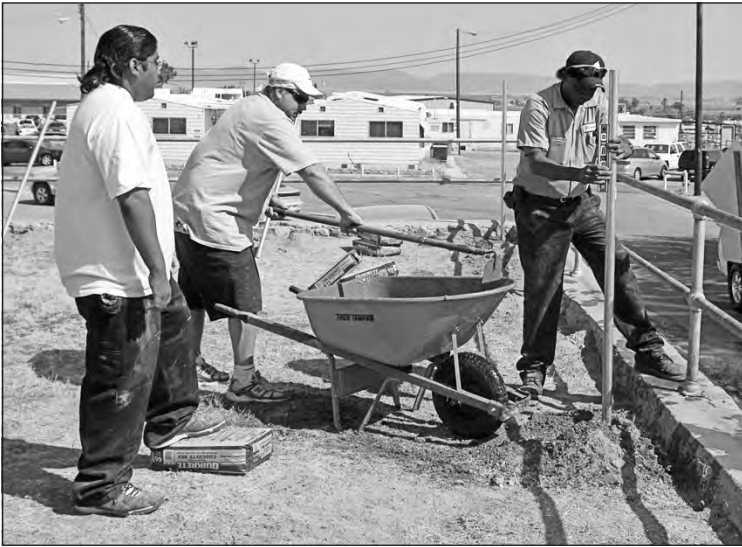
Wayne Chaipos, Jr. watches as Jeff Hagadus mixes concrete and Lonnie Gilmore checks the level of a fence post before the team pours the footing for it.
