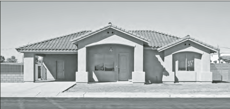
Rental homes in the new subdivision can also be had with a Spanish tile roof. All of the homes have a substantial appearance, as nice as any upper income ownership home in the Yuma/El Centro market.
