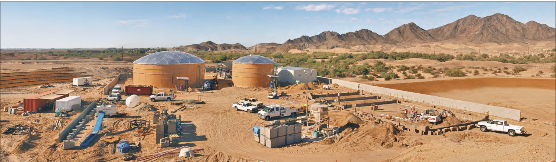
The Casino♠Resort's water treatment plant is located on the back side of a ridge to the south of the main complex. It has two groundwater wells just inside the east wall, an 850,000-gallon storage tank to hold fresh well water and provide water pressure, as well as a smaller tank to capture the water returned for treatment from the drains at the Casino♠Resort. To the east (on the other side of the wall on the right) is the 1,485,139 square foot retention basin which will hold stormwater and excess treated water for irrigation.
