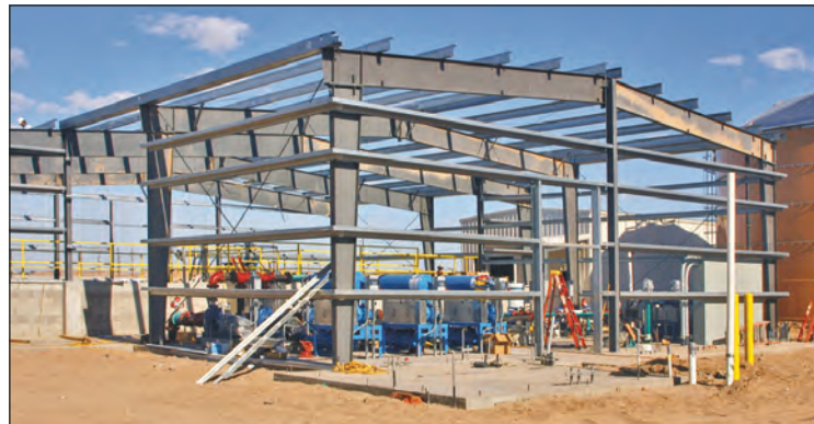
The pump house (above and below) for the state of the art water treatment facility just south of the Casino♠Resort is well on its way to being finished. The settling tanks are in, and the storage and water return tanks have also been completed.
