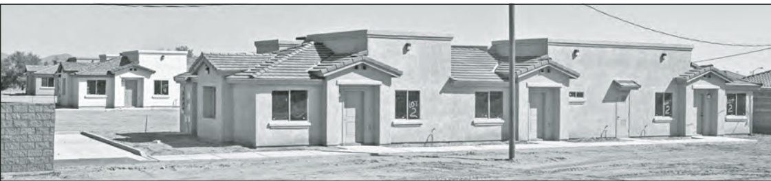
Three triplexes of apartments are also finished, awaiting only landscaping before tenants move in later this fall. Each unit has its own paved parking and a back porch area with a sliding glass door.
