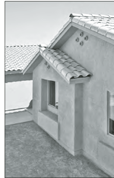
Every home being built abounds in interesting architectural details, such as the extended wall with its own peaked roof seen surrounding the front bedroom window of this unit. Note also the round vents arranged in a diamond pattern.
