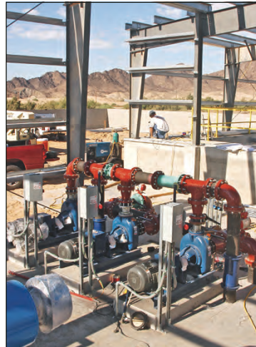
The pump house (above and below) for the state of the art water treatment facility just south of the Casino♠Resort is well on its way to being finished. The settling tanks are in, and the storage and water return tanks have also been completed.
