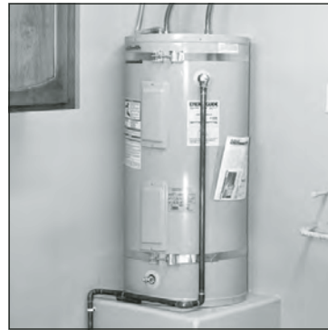
Water heaters are mounted up off the floor and secured in place to meet seismic standards.
