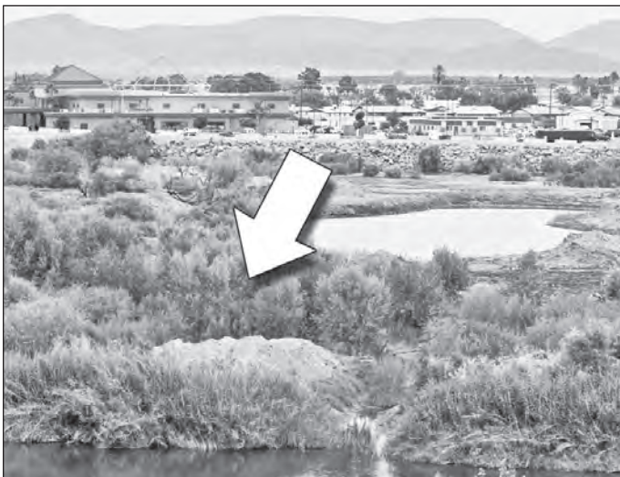
From Prison Hill, the location of the future Elder Village can be seen where a mound of dirt has been placed in the area for fill.
