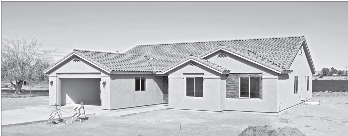
The first of the ownership homes is a "scattered homesites" 4 bedroom house just off First Street in Winterhaven. It was nearly complete just after Valentine's Day in February, when this photo was taken. QUECHAN NEWS Photo by William Isbell
