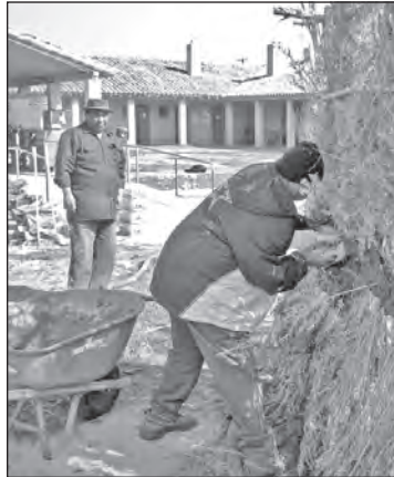
Dana Miller watches as Ivan Valisto applies some mud to the back wall of the hut, once the crowds have left and they can finish the structure.
