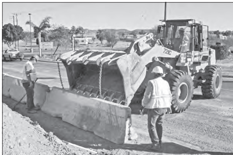
Concrete barricades were placed between the hill and the roadway afterwards to prevent any falling rocks from rolling down into traffic at some later date. Photos by William Isbell for The QUECHAN NEWS
