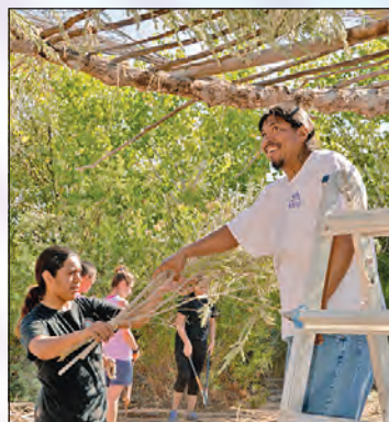
Valencia Gilbert, Laura Arriaga, and Brenda Acosta spent most the morning trimming and bundling fresh cut arrow weed, used to cover the roofs of all the buildings at the Elder Village. That's Orlando Jefferson handing off more roof thatching to Frank Venegas. Kilik Waters also pitched in with bundling and tying arrow weed, once he finished trimming the trees. The north half of the shade structure roof was all re-thatched in time for everyone to take a break at 10:00 AM to hear Lorey's historical/environmental lecture.
