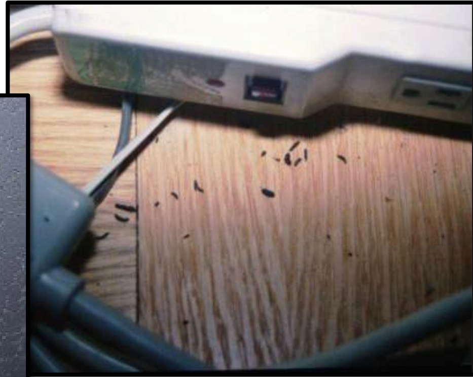
Mouse droppings by a power strip
